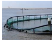
This cage's handrail tube collapses.
